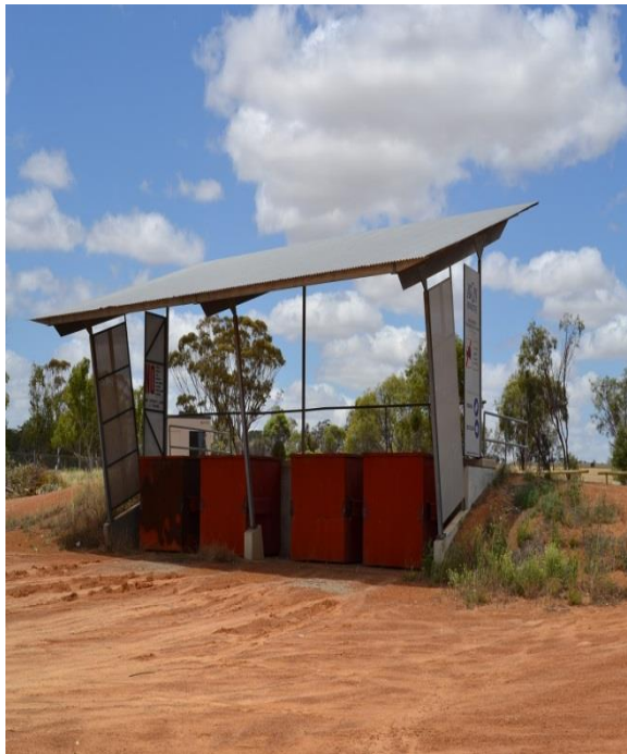
Meckering Transfer station
